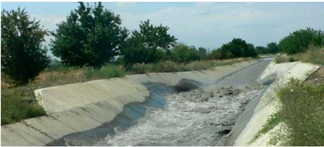
The Khanarc Canal was designed so that water flows under gravity, saving the expense of pumping.
